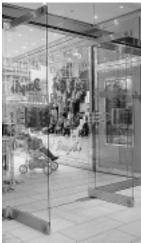
Example of an HSW-G system Fully glazed with door rails
